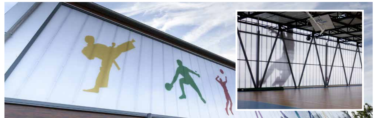
Nurcery School, France | Glazing: Danpalon® Printed, 16mm | Architect: Weber et Albrech
