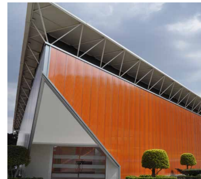
Cafeteria Unitec Atizapan, Mexico | Glazing: Danpalon 3DLITE. Danpal 16mm
