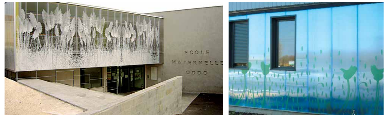
Odde Nursery School, Marseille, France Glazing: Danpalon® Printed, 16mm | Architect: Camille Richard Lenoble
