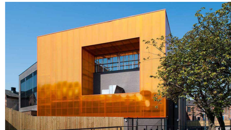
Blackburn Youth Zone Center, United Kingdom Danpal® Single System 16mm | Architect: Jackson Teese
