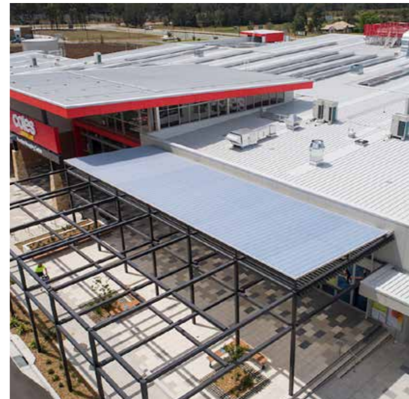
Coles Shopping Village Huntlee, Australia Architect: EJE Architecture
